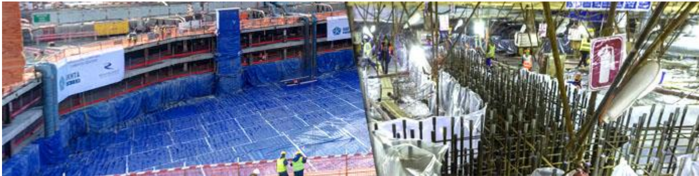
The bottom slab of the box shaped foundation
